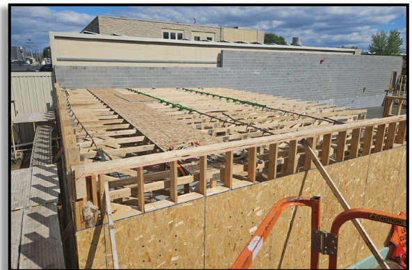
Roof Truss Framing Progress
