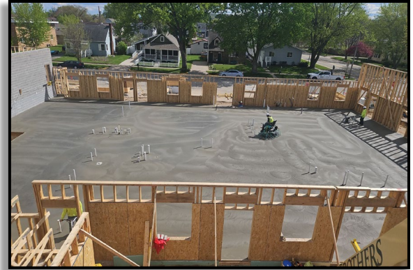
Concrete Floors Complete
