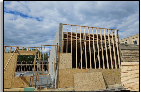
Wall Framing Progress
